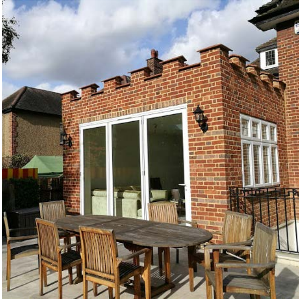
(No.1 Seaforth Gardens' rear extension)
